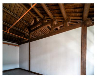
Figure 19. The traditional Chinese roof-truss system of "Tianbaoli" townhouses.
