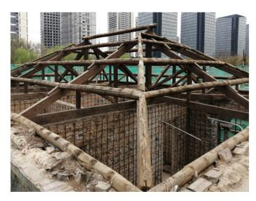
Figure 20. The Western triangular roof-truss system of the Priest's Residence.
