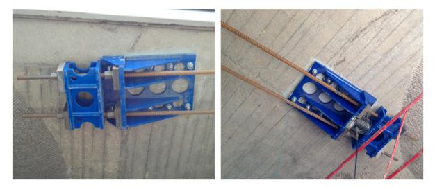
Figure 22. Passive (left) and active (right) anchorages.
