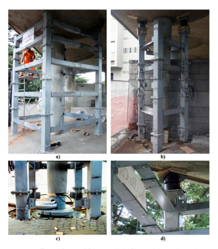
**Figure 10.** Different lifting steel frames: (a,b) the four- and three-columned ones, respectively, (c) base detail of the lifting frame, and (d) adjustment of the hydraulic jack head on the inclined surface of the mushroom column.
