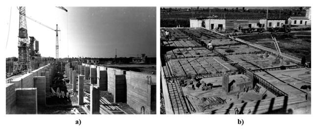
**Figure 6.** Archive photos of the Reinforced Concrete (RC) box at the basement: (**a**) before and (**b**) after the realization of the slab (note that the clay blocks, with which the slab is made, are clearly visible).
