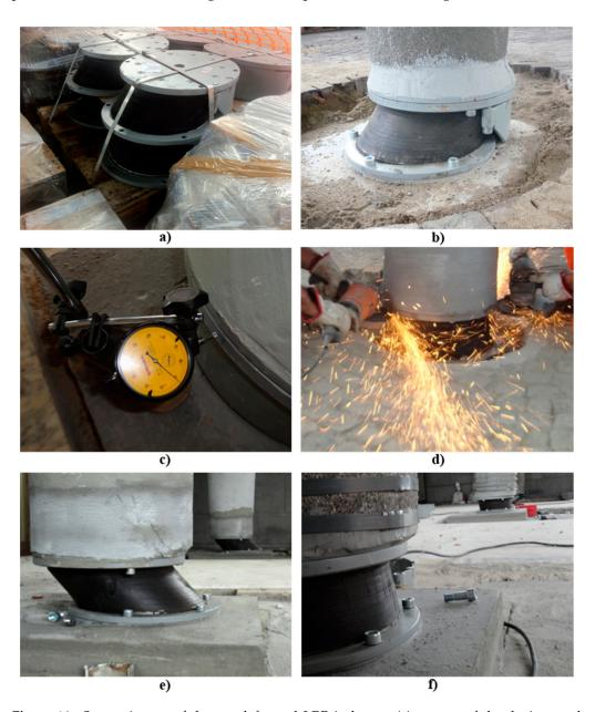
**Figure 14.** Some pictures of the pre-deformed LRB isolators: (a) storage of the devices at the construction yard; (b) pre-deformed LRB installed under the column; (c) installation of the high precision displacement transducer; (d) removal of the temporary constraint; LRB device at (e) the beginning, and at (f) the end of the re-centering operations.
