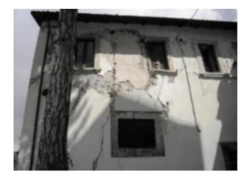
Figure 1. Damage concentrated at the irregularities on masonry buildings [28].
