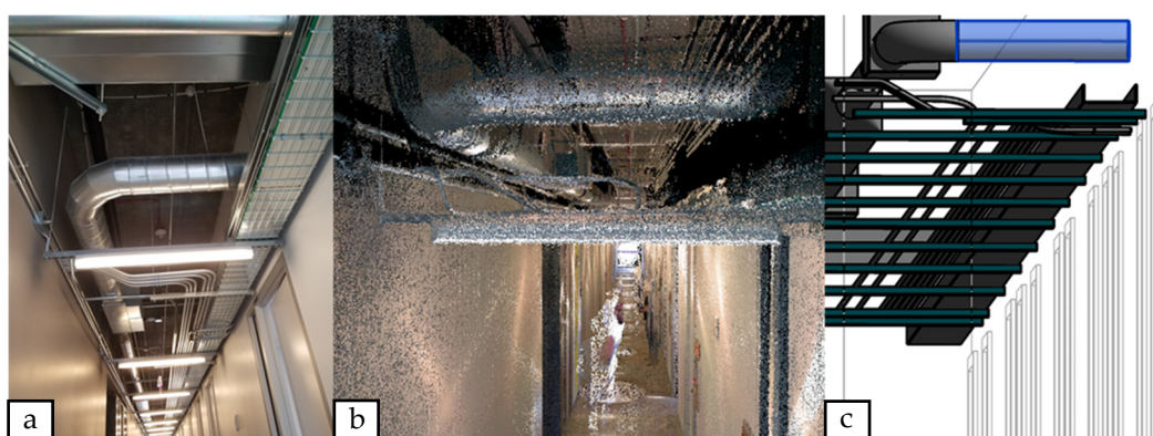
Figure 1. (a) Photograph of the built environment, (b) laser scan, and (c) resultant model. Approximate test area physical dimensions are 5 ft. wide by 25 ft. long.
