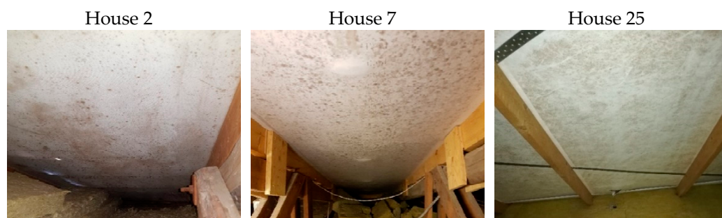
Figure 20. Mould growth in the attics of three test houses, namely houses 2, 7 and 25.
