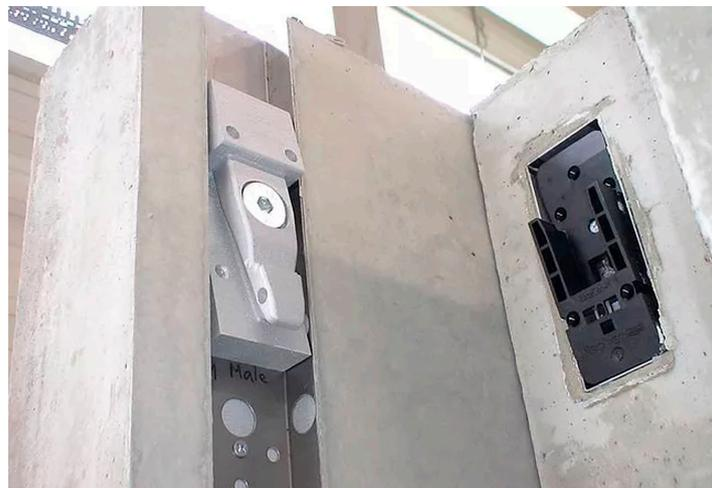
**Figure 9.** UNICON connecting system by Munitec GmbH [39].
