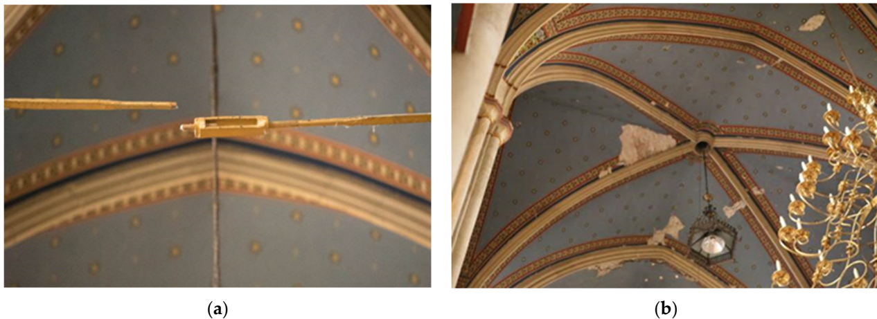
Figure 1. Cathedral of the Assumption of Mary, Zagreb: (a) Fractured tie rod after its load bearing capacity was reached (b) Damaged vaults after the March 22nd 2020 Zagreb earthquake.
