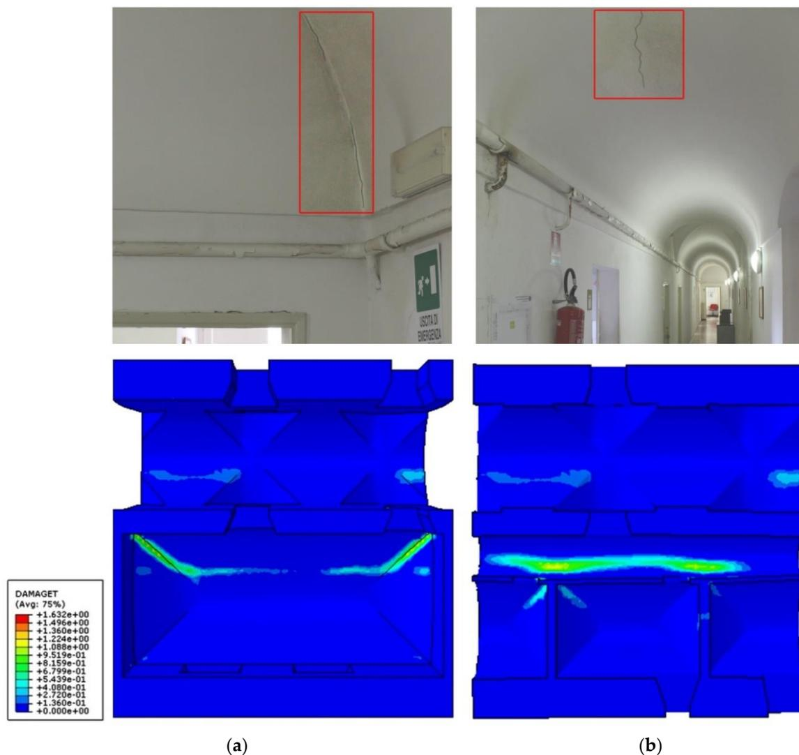
**Figure 15.** Comparison between the damage survey and the crack pattern at the vaults' intrados coming from the finite element analysis for inwards seismic action: (a) ground floor; (b) mezzanine floor. The damages are between 0 and 1.6.
