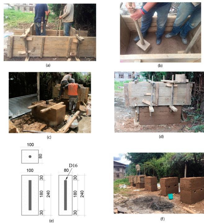
**Figure 1.** Rammed earth (RE) specimen construction: (a) formwork placement for the lower RE block; (b) ramming of earth soil, (c) insertion of the reinforced concrete (RC) dowel, (d) formwork placement for the upper RE block, (e) details of RC dowel, (f) completed rammed earth specimens.
