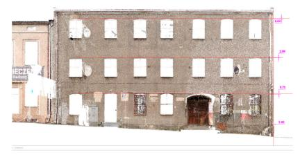
**Figure 10.** Outside view of the building made using TLS in Autocad 2015—Front wall with measured deformation [cm].
