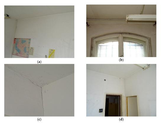
**Figure 4.** Interior damages: (**a**) wall cracks; (**b**) damages near the masonry arch lintel; (**c**) wall corner damages; (**d**) cracks near the ceiling base.
