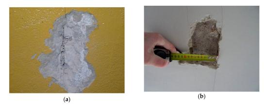
**Figure 5.** Uncovered main structure elements: (**a**) vertical crack of the brick wall; (**b**) measurement of uncovered steel beam.
