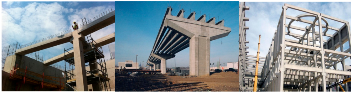
Figure 3. Examples of simply supported reinforced concrete beams of T, I, and rectangular cross-sections used in building structures.
