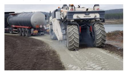
**Figure 4.** Preparation of the recycled mixture under field conditions using the "in situ" method [P. Buczyński].
