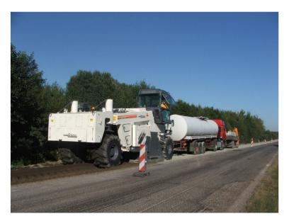
**Figure 1.** Manufacturing of the bitumen emulsion (MCE) mixture using the "in-place" method. [J. Krasowski].
