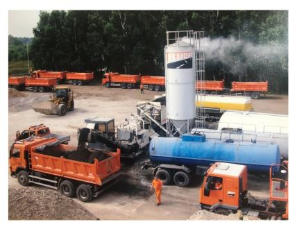
Figure 2. Performing of the MCE mixture using the "in-place" method. [J. Krasowski].
