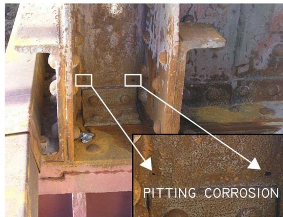
**Figure 1.** Example of pitting corrosion in a structural component.
