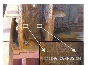
Figure 1. Example of pitting corrosion in a structural component.
