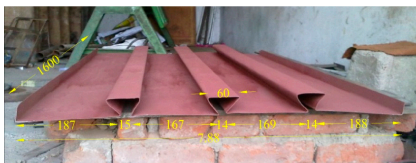
Figure 3. Dovetailed or re-entrant profiled sheet (All dimensions are in mm).
