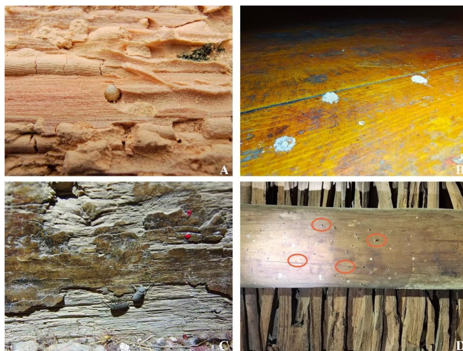
Figure 8. Habitat and biological characteristics of L. potala . (A) Larva and larval galleries within wooden structural components (from [12], reproduced with permission from the copyright holder, ©Magnolia Press). (B). Frass accumulated at the gallery opening. (C) Adult active near wooden structural components. (D) Dead adult blocking the gallery opening (indicated by red circles).
