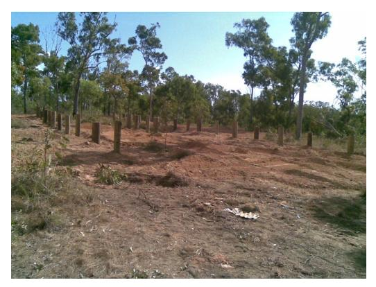
Figure 4. Power pole stubs installed at experimental site.
