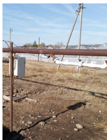
Figure 16. The automatic reagentless geothermal water treatment system control cabinet.
