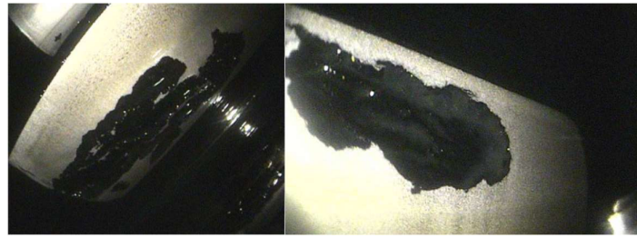
Figure 4. Pitting and spalling on the pinion gear mounted on the HSS.
