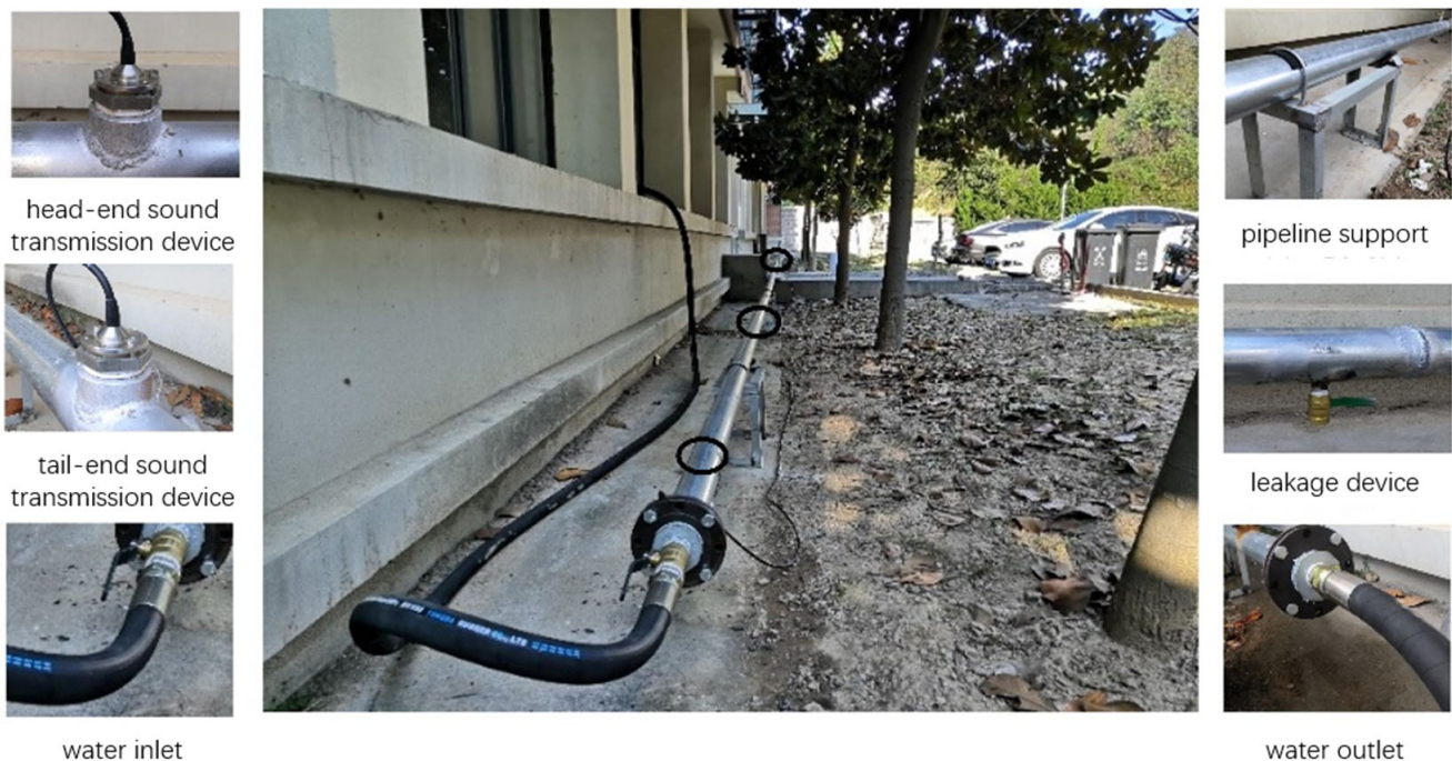
Figure 6. Testing pipeline site.
