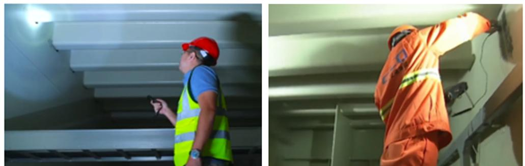
**Figure 1.** Manual inspection inside the SBG of a bridge.
