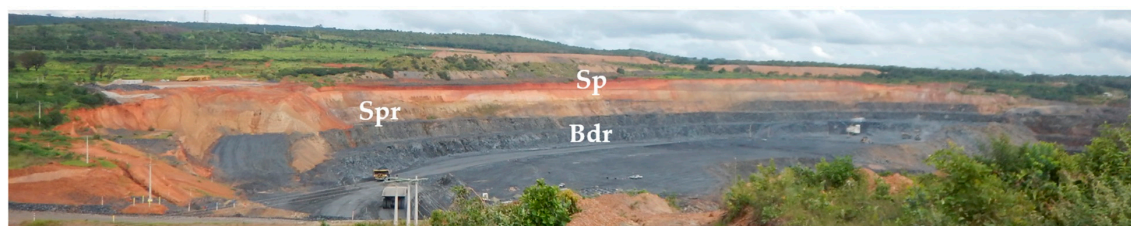
Figure 5. Weathering profile exposed at the southwestern part of the Paracatu mine. The vertical profile shows a red saprolite (sp) transitioning downwards into saprock (spr) and fresh bedrock (bdr). Pit bench height is 12.5 m. The panoramic view looks north-north-east (NNE).
