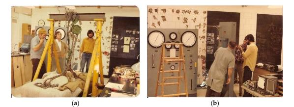
**Figure 1.** Installation of Harwood 500-ton press and girdle-anvil apparatus in 1977. (**a**) Bob and technician Tony Vidmar contemplating how to bring the press to upright position; (**b**) Al Catalano (machinist extraordinaire) and Alan Major from ANU with Tony Vidmar checking hydraulic connections to press.
