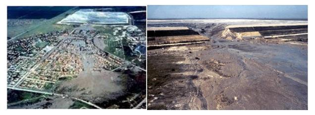
Figure 5. Failure of the Merriespruit tailings dam in South Africa, due to overtopping and flow liquefaction [5].
