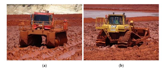
Figure 19. Farming red mud, by (a) a scroller, and (b) bulldozing with a D6 Swamp Dozer.
