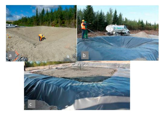
**Figure 3.** (**a**,**b**) sand and geomembrane installation, respectively, and (**c**) filling the control cell with reactive tailings.
