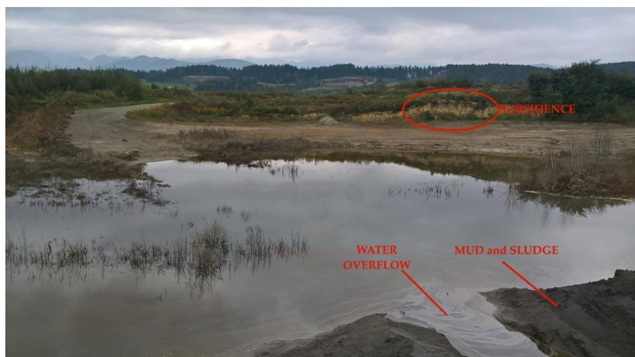
**Figure 8.** Situation form site, visual presentation of subsidence, overflowing of water, and presence of mud and sludge.
