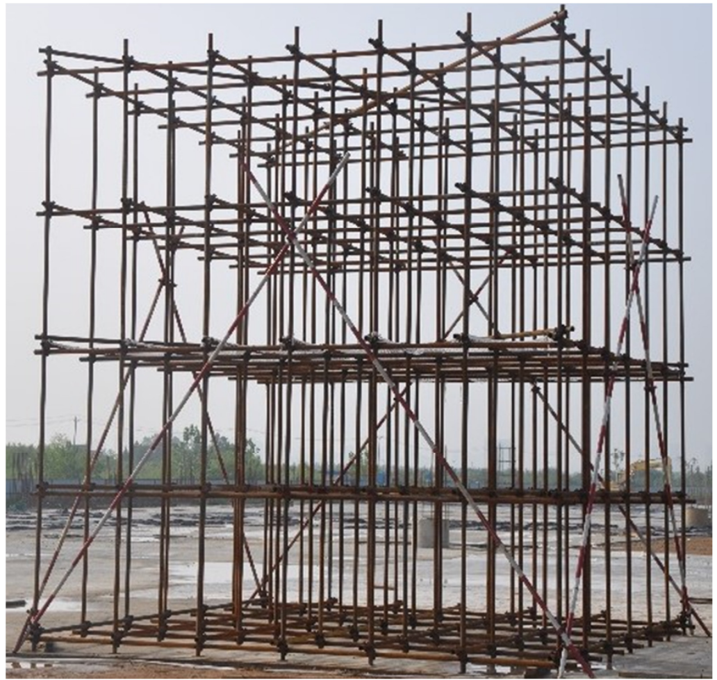
Figure 20. The photography of the high formwork.
