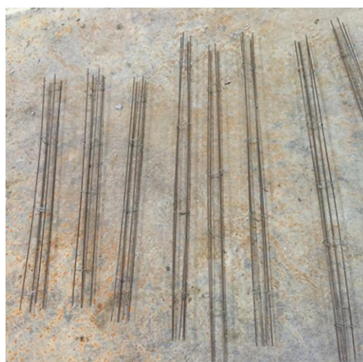
Figure 5. Reinforcement cages.
