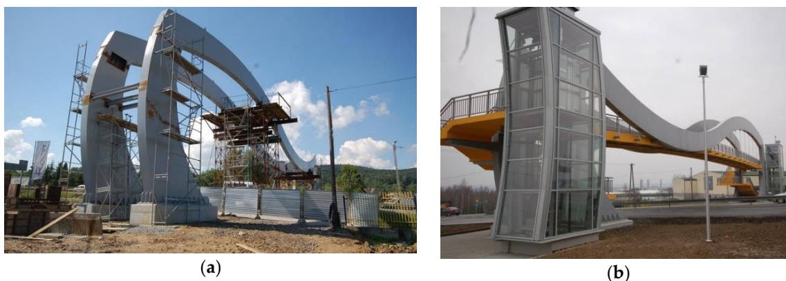
Figure 3. The footbridge structure: (a) steel frame during the montage, (b) the footbridge after assembly [18].
