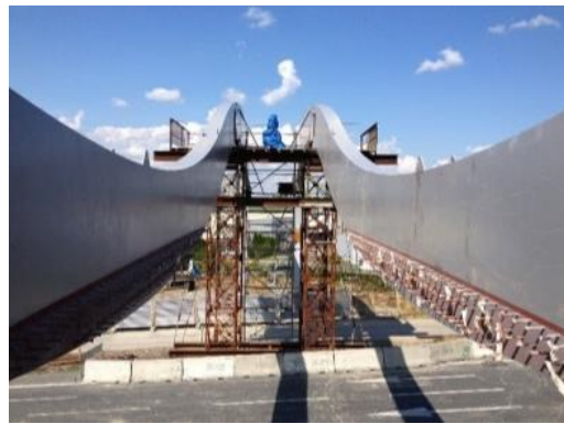
Figure 5. The structural layout of the pedestrian bridge over the national expressway located in Jawornik (Southern Poland) [18]: (a) cross-section, (b) steel frames of the footbridge.
