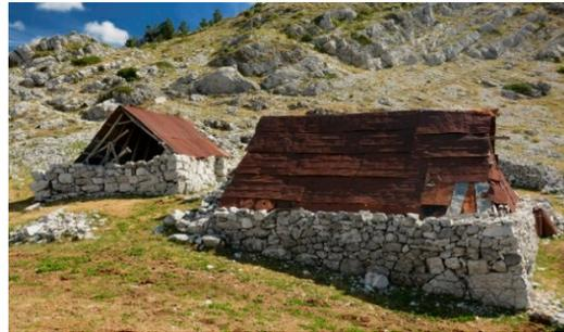
**Figure 31.** Glada's roof made of the tin barrels—Koštica, Kotski katun, photo: I. Laković.
