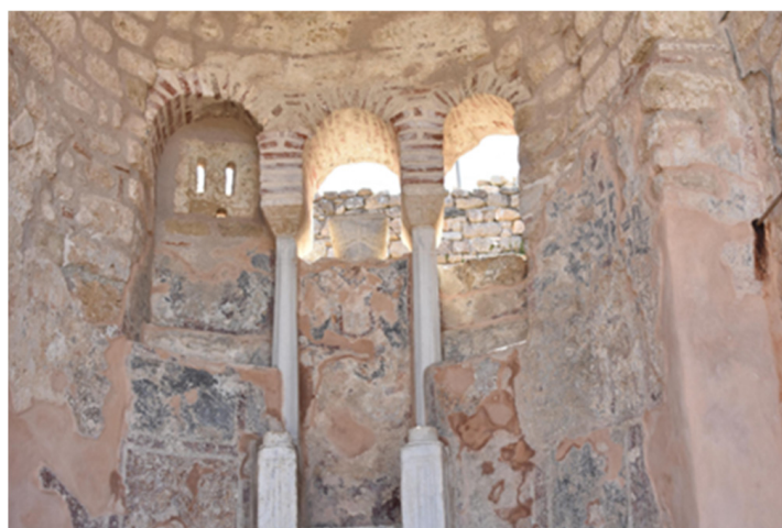
Figure 4. Integration of local geomaterials in Chora Castle's masonry, featuring ancient marble spolia, porous Quaternary tufa, and traditional schist-based 'melagi' mortar.
