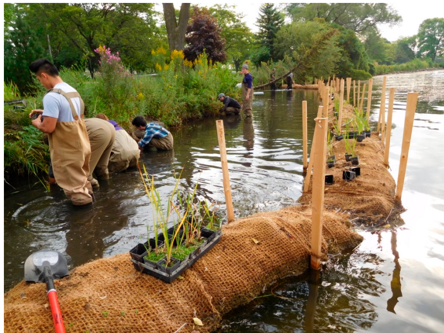
Figure 5. Brush bundle wave barriers (buckthorn wrapped in coir fabric) in place along the northern shore of the eastern basin of Lake Winona, anchored in place with wooden stakes (stakes were shortened later). Volunteers are shown planting emergent aquatic macrophytes to stabilize the shoreline.
