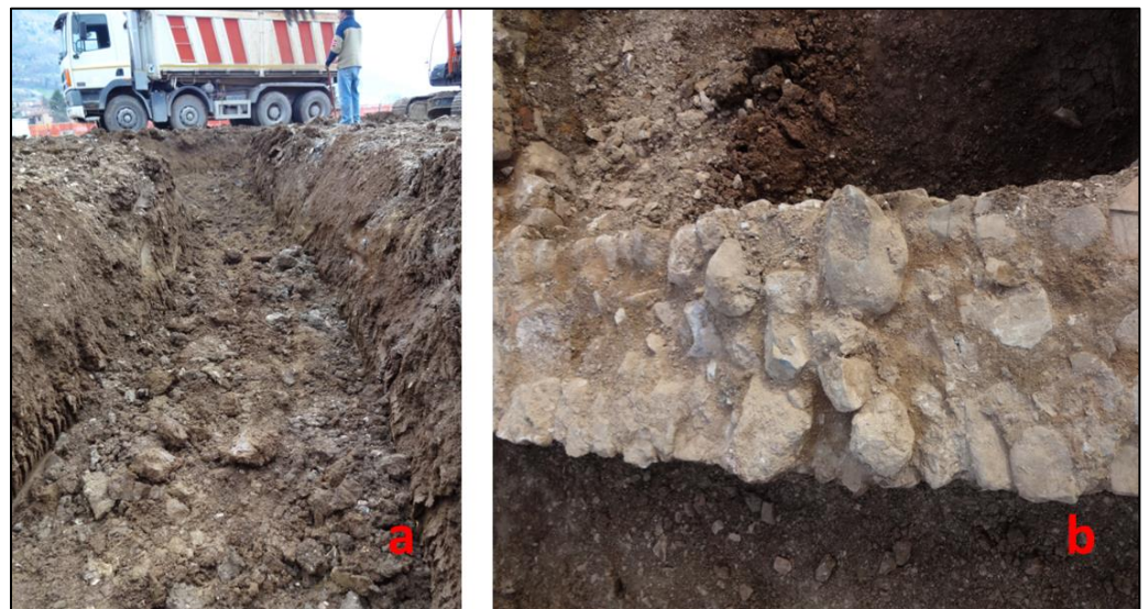
Figure 8. (a) The trench made during the excavation of the building in Figure 7; (b) pebbles of clear fluvial origin used to build the artifact.
