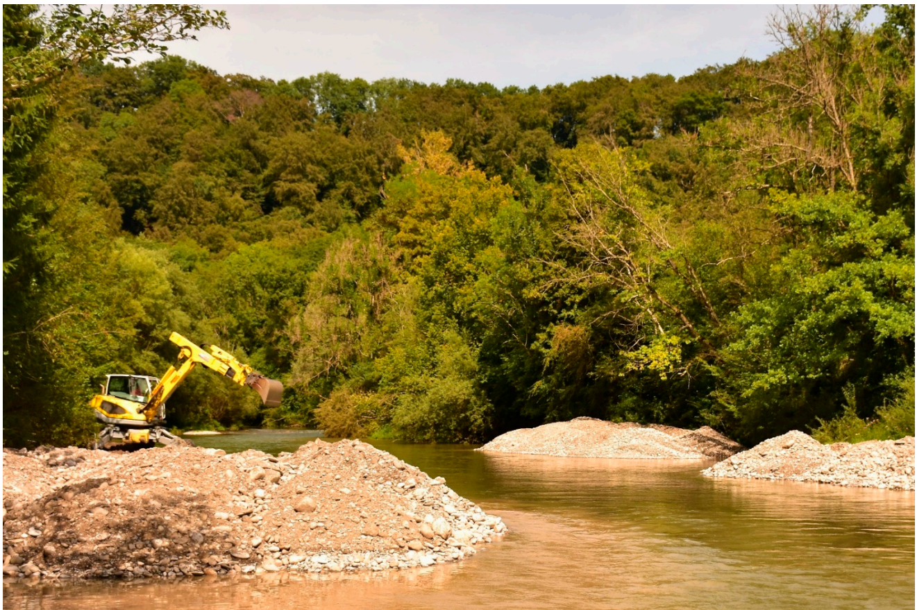
Figure 3. Installation of in-channel stockpiles at the residual flow section of the Sarine River, downstream of Rossens Dam, Switzerland, in 2016. About 1000 m 3 of an alluvial sediment mixture from the adjacent floodplain were injected and coupled with an artificial flood to improve the downstream riverbed structure and increase habitat diversity.
