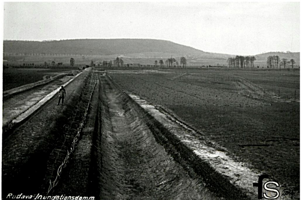
**Figure 5.** View of the levee and inundation channel from the side of the Rudawa millrace. Archival photograph from 1915, from the author's collection.
