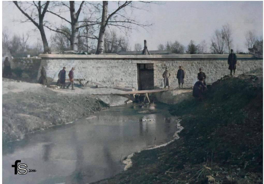
**Figure 4.** View of the damming wall of the *Wilga-Schleuße* fortress weir, seen from the side of the inundation area. Archival photograph from 1915. From the author's collection.
