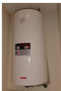
Figure 4. Example of an electrical water heater used for the shower.
