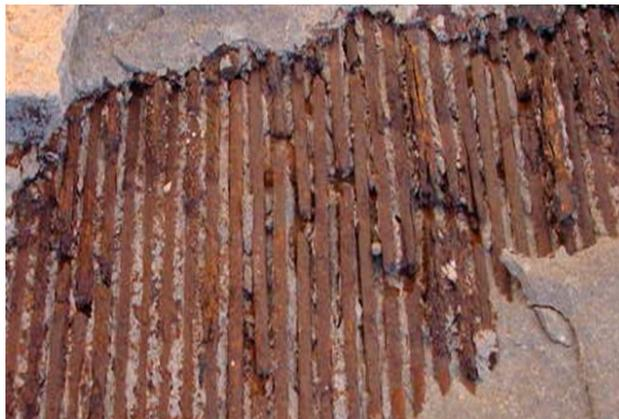
**Figure 4.** Distressed area of a PCCP.
