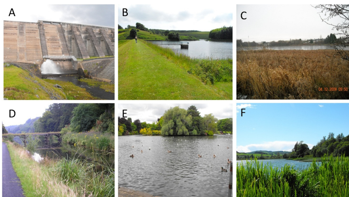
Figure 2. Typical examples for six different types of sustainable flood retention basins. (A): Hydraulic Flood Retention Basin; (B): Traditional Flood Retention Basin; (C): Sustainable Flood Retention Wetland; (D): Aesthetic Flood Treatment Wetland; (E): Integrated Flood Retention Wetland; (F): Natural Flood Retention Wetland.
