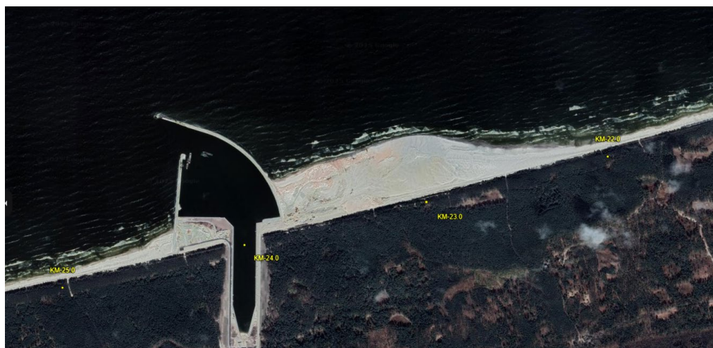
Figure 4. A view of the Vistula Spit Channel port, constructed in 2022. A western breakwater with a length of 568 m; an eastern breakwater extending to 1014 m. Both structures are impermeable breakwaters with a core, armored on the seaward side with Xbloc and XblocPlus units. Large-scale artificial beach nourishment project, 2.2 mln m 3 deployed.
