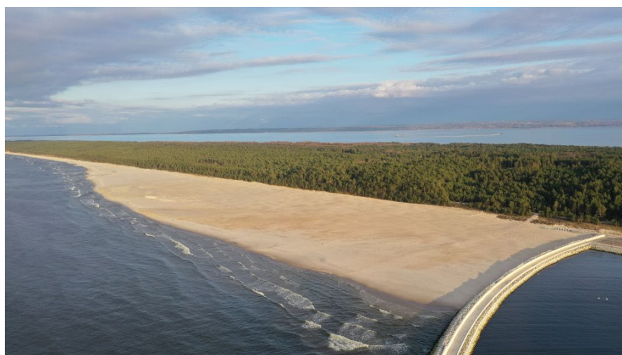
Figure 5. View of the large-scale artificial beach nourishment project (2.2 mln m 3 of sand) and part of the eastern breakwater. Picture taken in 2022.
