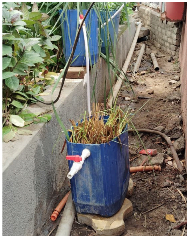
Figure 5. Chrysopogon zizanioides (vetiver grass) established in Container 2 (second stage) of the MTBRCW system.
