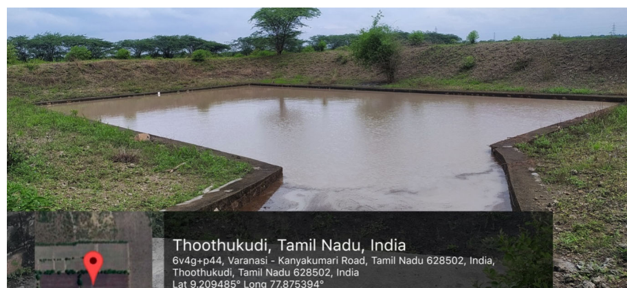
Figure 8. Concrete-lined RWH pond.
