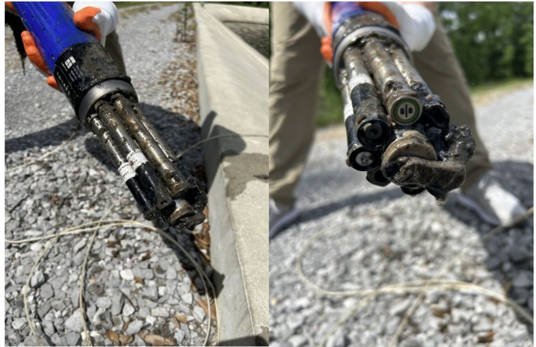
Figure 2. Bimonthly maintenance check for the primary settling pond S1 to show fouling and central wiper blade cleaning efficiency.
