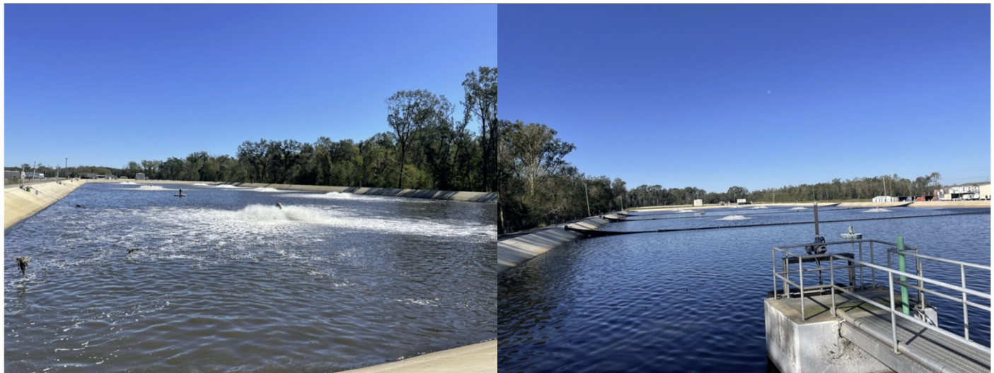
Figure 1. The primary settling pond (left) with the 25-horsepower aerator and the secondary treatment pond (right) with the gravity-fed outfall basin. The S1 sampling location is stationed to the sidewall of the pond near a 25-horsepower aerator, while the S2 sampling location is on the back right corner of the concrete basin in the green vertical pipe.
