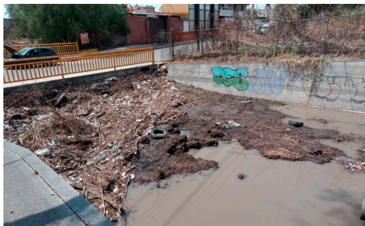
Figure 4. Photograph of sediment and material deposition on the vehicular bridge located downstream of the Sector Popular natural wetland as a consequence of traditional management (March 2023).
