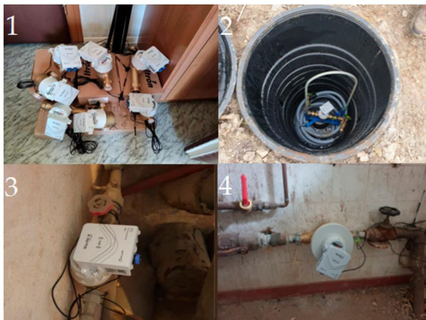
**Figure 2.** The figure shows photos of the field research: (1). measuring sets ready for installation; (2). a measuring set installed on the connection of a single-family house; (3). a measuring set—water meter DN20 mounted on the connection of a multi-family house; (4). a measuring set—water meter DN40 mounted on the connection of a multi-family house.
