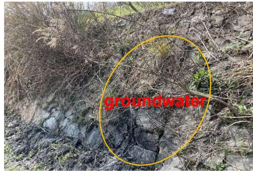
**Figure 3.** A small amount of groundwater seeps from the retaining wall.
