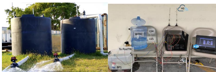
Figure 5. The prototype of the automatic remotely water releasing structure.
