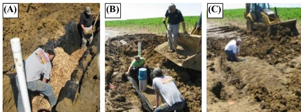
**Figure A1.** Installation of an ATI. (A) A layer of woodchips is placed in a trench over an existing drain tile. (B) Pea gravel is placed over the woodchips. (C) The gravel is slightly mounded.
