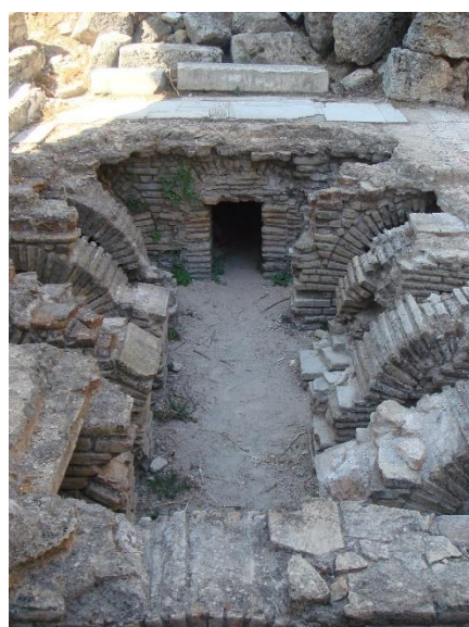
Figure 19. Hypocaust of the hot baths in Perge. The picture was taken by one of the authors [72].
