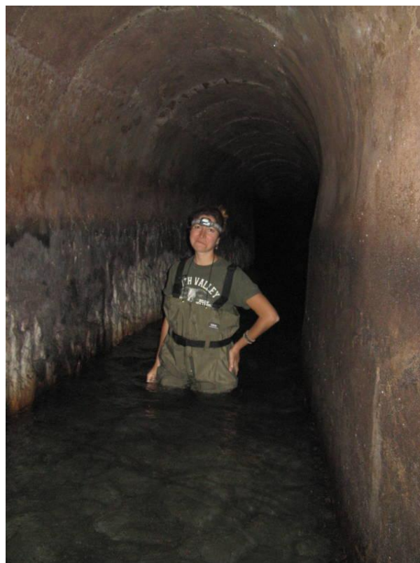
Figure 11. The AQUA VIRGO in Rome is a Roman aqueduct that still transports approximately 1 m 3 /s ( Photo Cees Passchier) [11].
