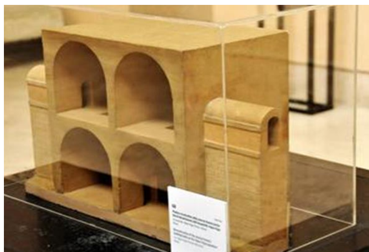
Figure 7. Model of the settling tanks (piscina limaria) on the aqueduct Virgo in Rome (Roman Civilization Museum in Rome, by permission of L. W. Mays).
