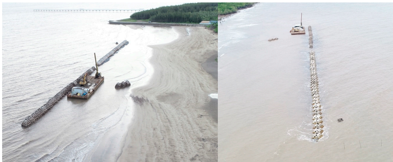
Figure 17. Wave breakwaters with PTPBW structure, which was designed on the basis of the present research results.
