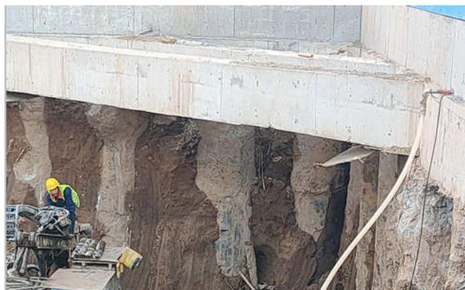
**Figure 4.** On-site construction of corner braces.
