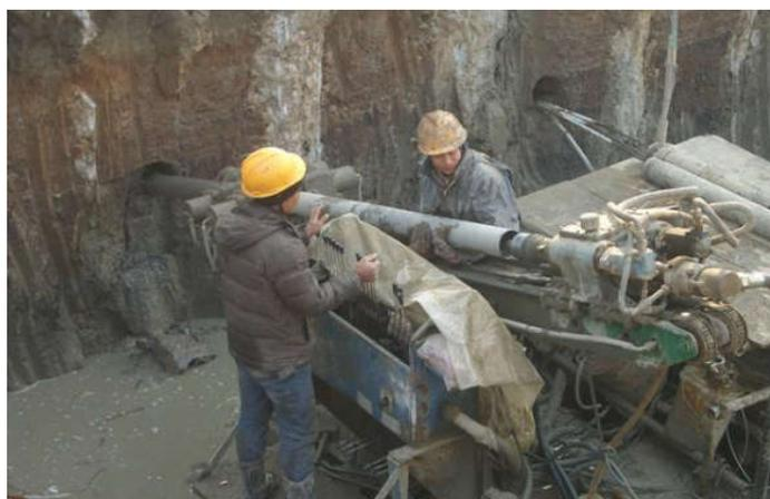
**Figure 3.** Drilling construction of anchor cable.
